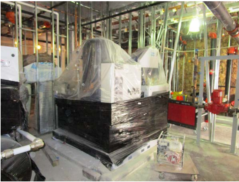
Photo 09 Level 01 – Air compressor unit set in place.
