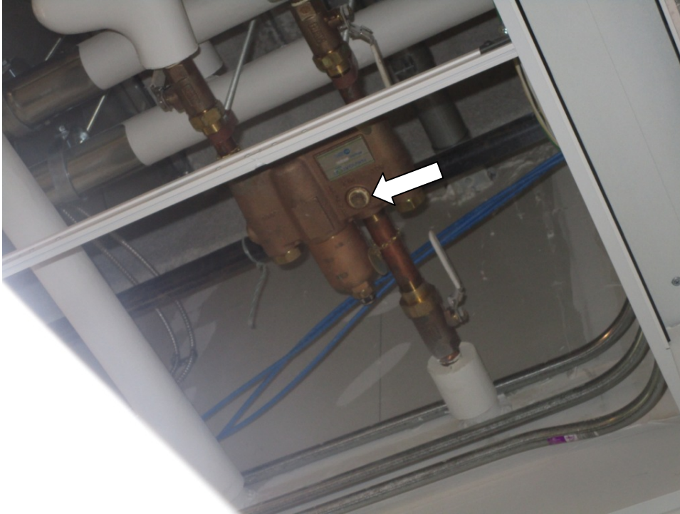
Photo 3-5 Ginny Harrison Organismal Biology Lab 378 – Missing thermometer gauge on TMV.
